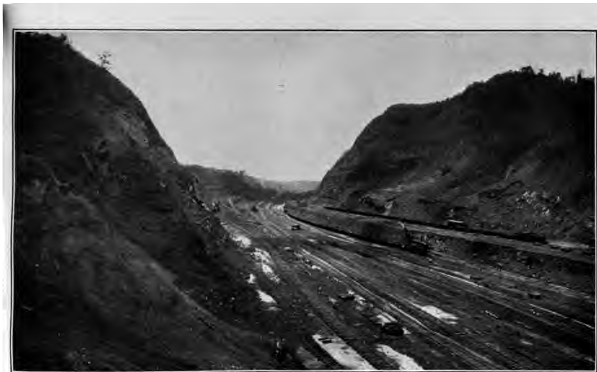
THE DEEPEST PART OF THE CULEBRA CUT.
